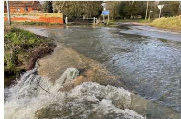
Flooding of "Church Hill" Road below Fields 4 & 5 17/01/21 observed by Claire Boulton
